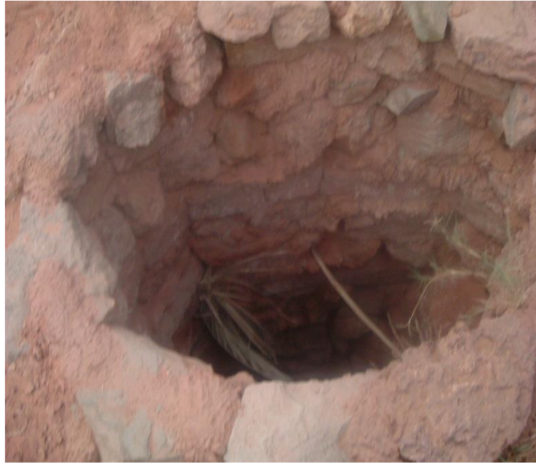
Fig. 3 An airshaft at the foggara of Gourara
